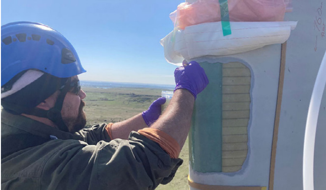
Once pressure belts were removed, NREL researchers David Barnes (above) and Ryan Beach and lead technician Mark Iverson set to work filling tiny holes in the leading edge of the blade left behind when the device's flyboards were removed. Image by Ryan Beach, NREL
