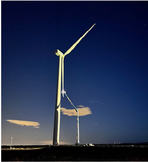
A technician on an extended aerial lift installs instrumentation on the wind turbine blade. Transitioning the wind turbine from upwind to downwind took weeks. Image by Pietro Bortolotti, NREL
